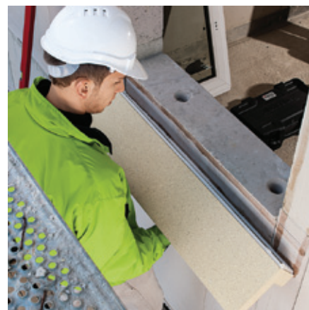
Obr. 6: Instalace L profilu PR010 na zdivo
